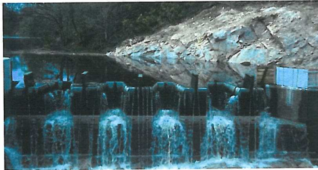
Photo of Saint Herbot Dam in France; 1.50m high labyrinth Fusegates
