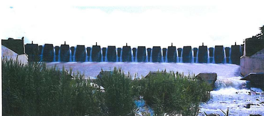
KAMUZU II DAM (MALAWI) - 5.0m high labyrinth Fusegates
